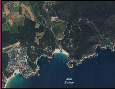
URBAN WASTEWATER TREATMENT PLANT PALAMÓS, GIRONA (SPAIN)
