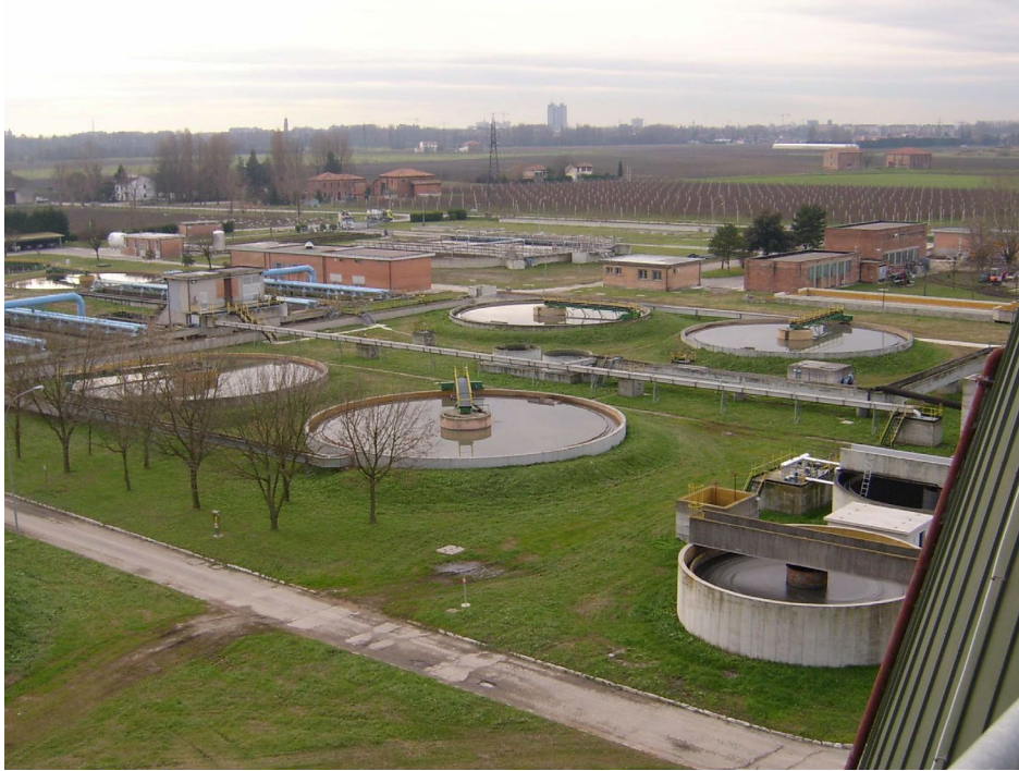
WWTP of Ferrara, Italy
